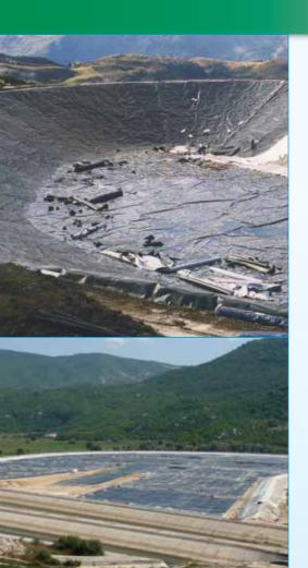
AGRU HDPE liners are used for the base sealing and the capping of landfill sites. Substances endangering a body of water are encapsuled and the flow of leachate is prevented. Due to the capping the infiltration of clean rain water is avoided.
