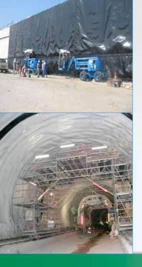
Due to the high level of flexibility the AGRU VLDPE tunnel liner guarantees a perfect adjustment to the tunnel structure, an easy installation and leak tight joints. The material has an excellent resistance to aggressive soil and mountain water.
