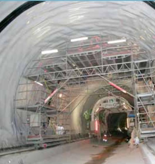
Due to the high level of flexibility the AGRU VLDPE tunnel liner guarantees a perfect adjustment to the tunnel structure, an easy installation and leak tight joints. The material has an excellent resistance to aggressive soil and mountain water.
