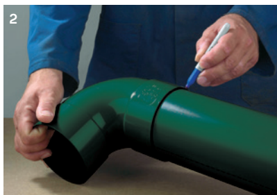
2 Mark the insertion depth
